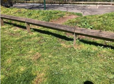
Galvanised rail fencing is proposed to improve resistance to vandalism to gain entry and increase durability over standard wooden posts. Tree planting to offer longer term protection would also be introduced in boundary areas currently open to entry.
